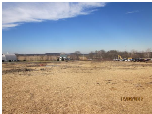
Lawn Road Yard. Temporary stabilization adequate in foreground, sparse in distance.
