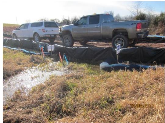
Timber bridge partially obstructing WW-T53-4001
