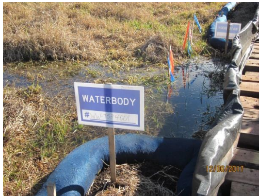
Timber bridge partially obstructing WW-T53-4001
