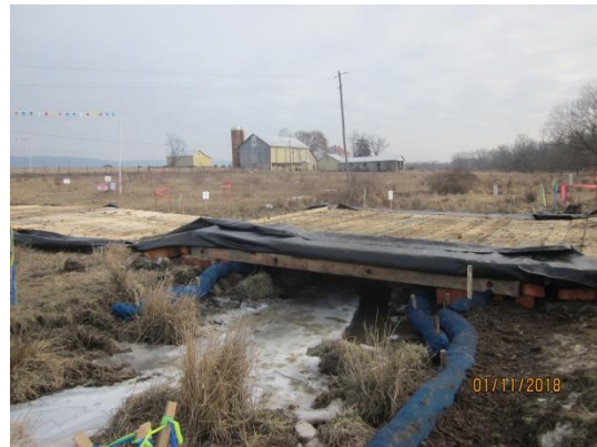
WW-T32-6001 east of Fort Swatara road. View facing downstream. Streambank disturbed by installation.
