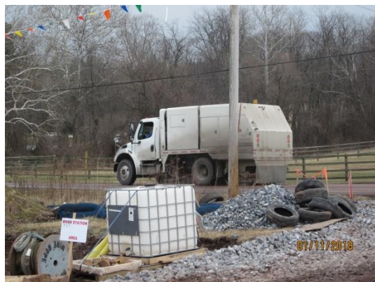
View facing southeast across Elizabethtown Road. Rock Construction Entrances clogged on both side of road. Small corner of clogged RCE visible in bottom right corner of photo.
