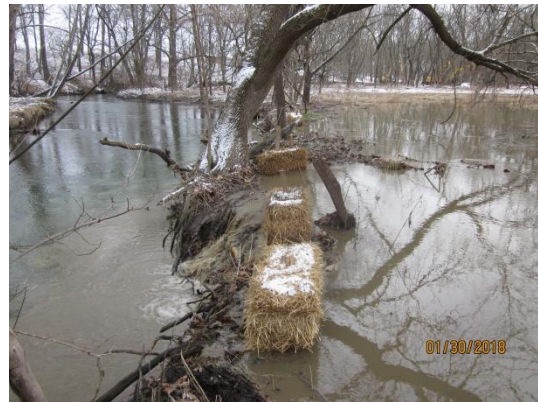
Bales between pump water discharge area and Clear Spring Road. Sediment laden water entering stream.
