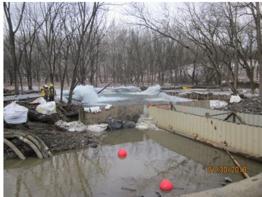
Flume and dam and pump in operation.
