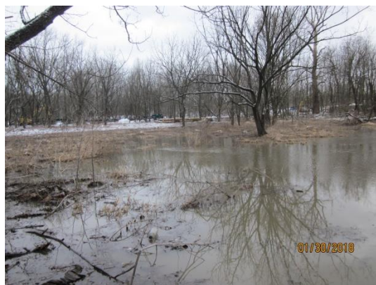
View standing on creek bank of ponding area between pump water filter bag and stream.
