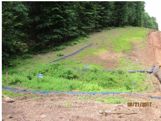
East of Beech Street. Sock installed at creek and wetlands.
