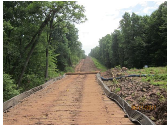
East of Beech Street. Timber mat with associated e&s installed.
