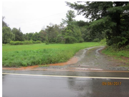
Sediment laden runoff leaving private drive along east side of SR 0117
