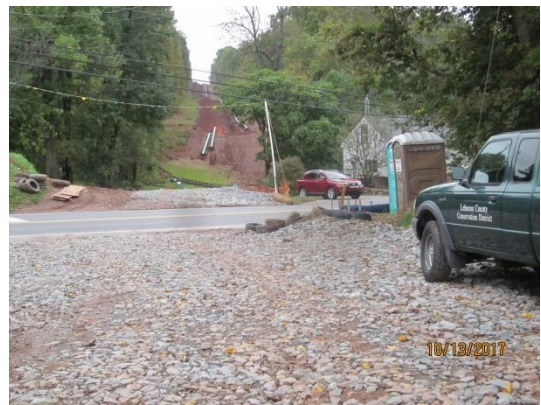
View of rce's looking west across SR 0117.
