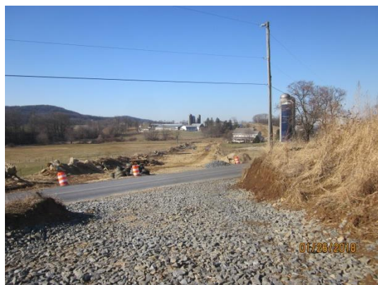
Well-constructed and maintained RCE on east side of Distillery Road.
